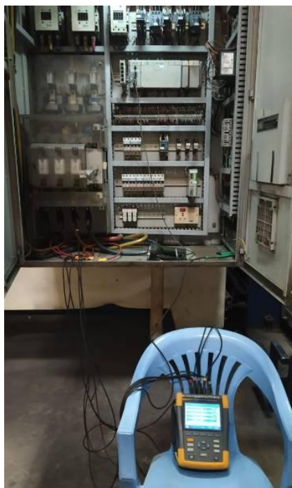
Figure 3 Connections of power analyzer
