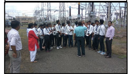
400KV Substation, Lonikand, Pune
